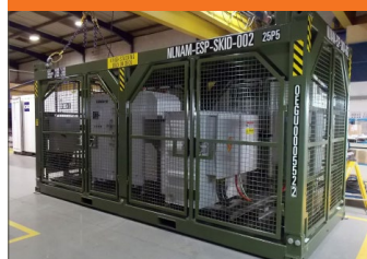
High Voltage Electrical Installation & Testing
