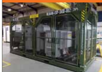
High Voltage Electrical Installation & Testing
