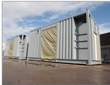
Modules fully painted to offshore specification and ready for outfitting
