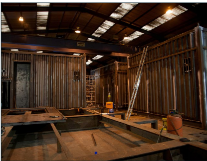
Fabrication of modules
