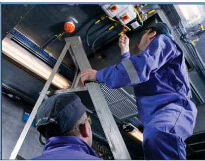
Outfitting work progressing
