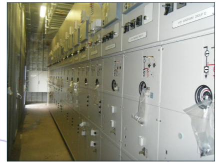
Electrical & instrumentation integration complete
