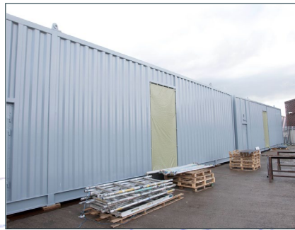
Modules positioned for equipment integration
