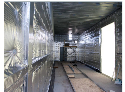
Initial outfitting of modules
