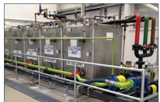
Figure 1 - Tank Washing System
